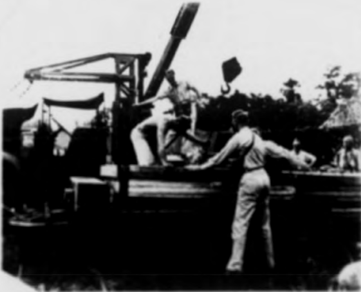
Lowering transport 170, 500 lb. of 3rd from point of explosion.
